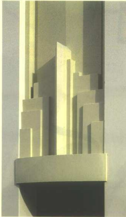
Sussan Building, West Melbourne (Formerly Symington Corset Factory), photo: David Thompson
